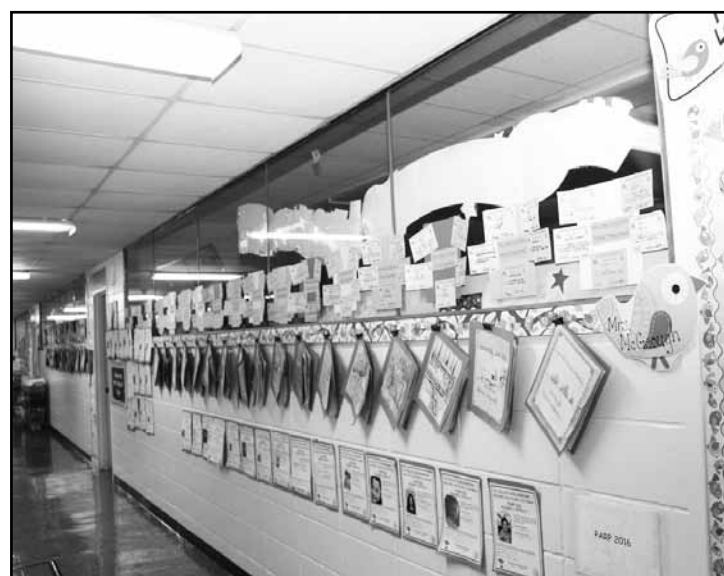
Many schools have partial glass walls that are not compliant with current building codes.
