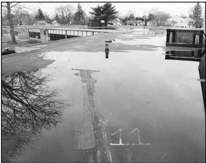
Ponding, which entails the collection of water, is a major problem for district roofs.
