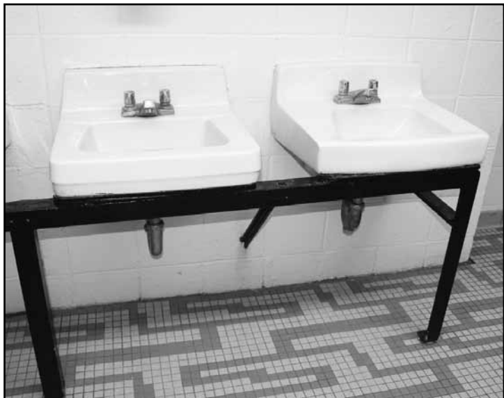
Bathroom sinks have been reinforced with framing to keep them from falling.
