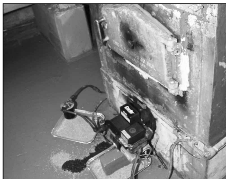
Burners are old, inefficient and have surpassed their intended life spans.
